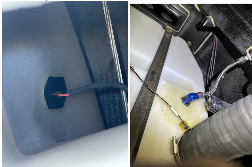
Figure 1. Examples of Leaks at Low Level Sensor (left) and Fuel Return Line (right)
